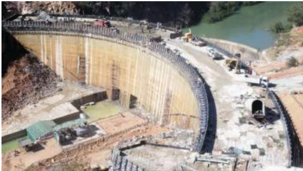
Construction of Gwayi-Shangani dam
