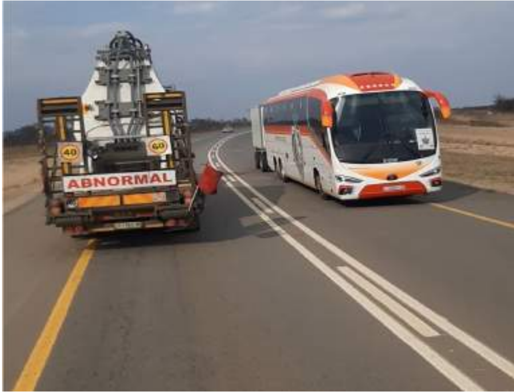
Completed Section of Harare-Masvingo-Beitbridge Road
