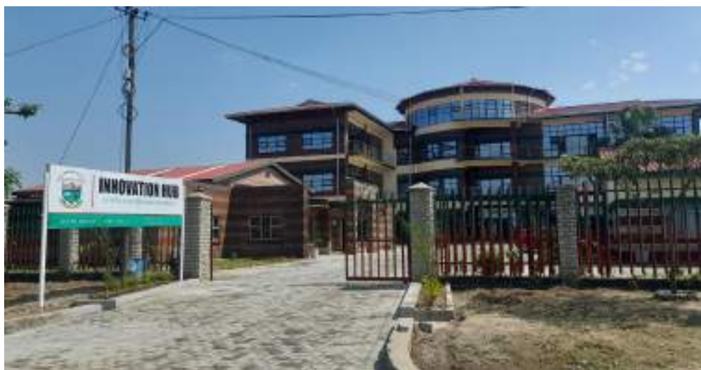
Completed Great Zimbabwe University Innovation Hub
