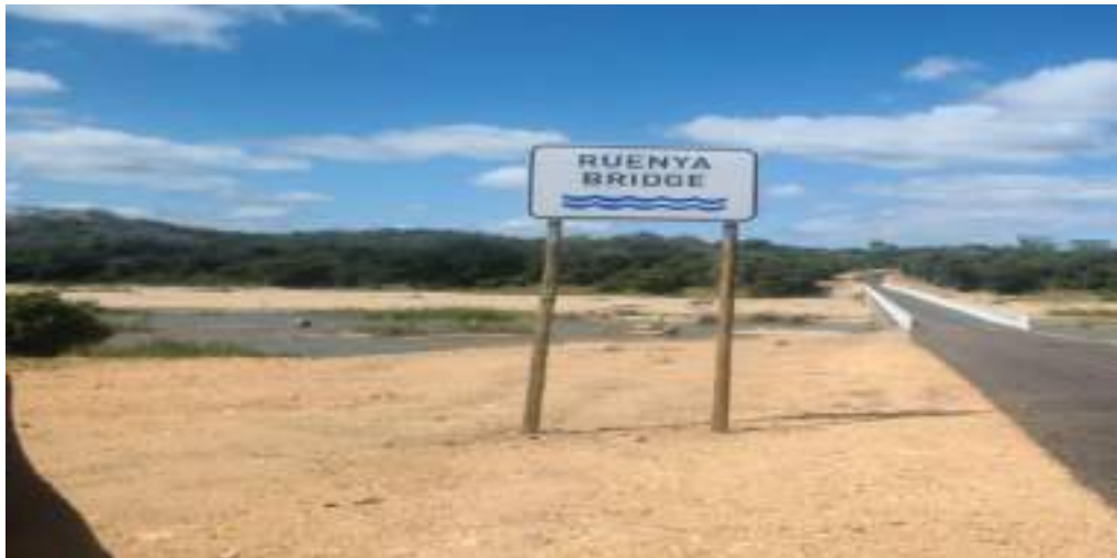
Ruenya Bridge, Nyanga
