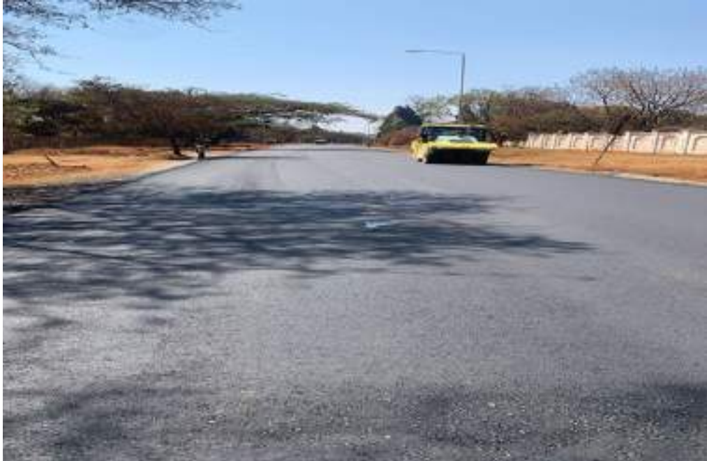
Rehabilitation of Alpes Road and Opened to Traffic, Harare
