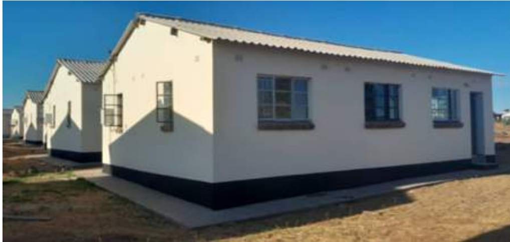
Construction of 19 Civil Servants Houses in Lupane, Matabeleland North Province
