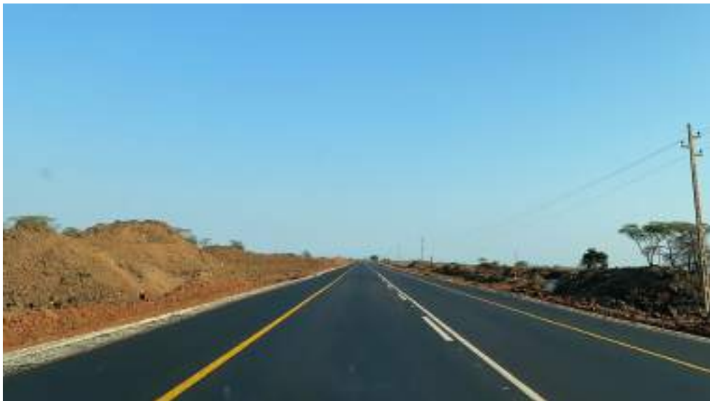
Completed Section of the Harare-Masvingo-Beitbridge Road
