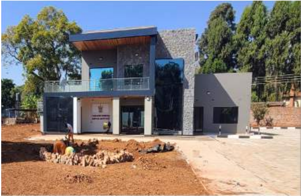
Renovated ZFSI front view (ZIMBABWE FOREIGN SERVICES INSTITUTE)
