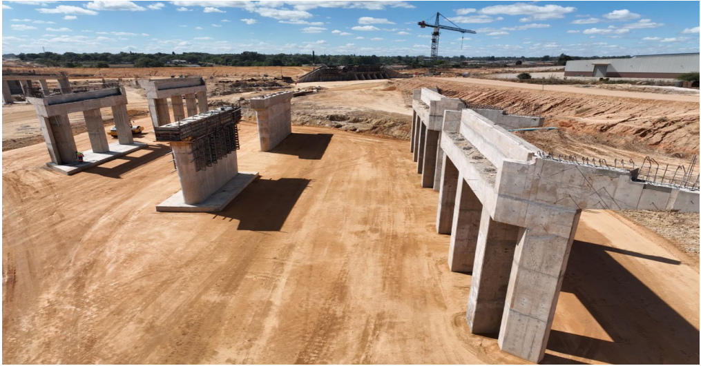
Aerial View of Mbudzi Interchange Bridges
