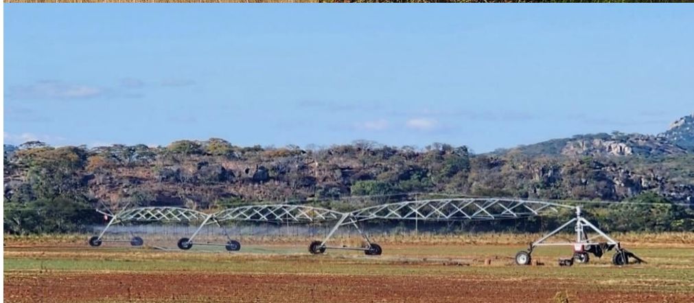
Manicaland State University of Applied Sciences Agro-Industrial and Innovation Park being fenced
