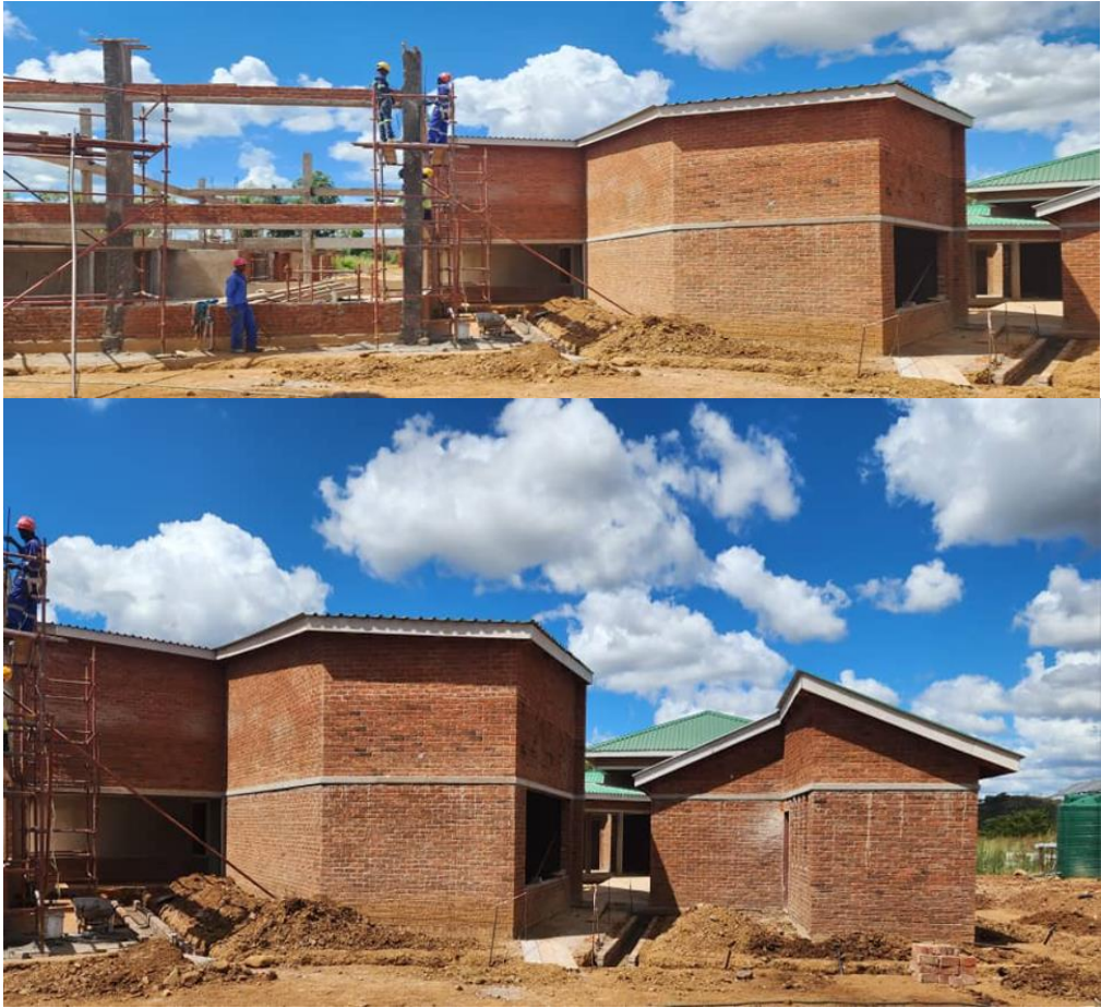
BUSE Kitchen and Dining Hall under Construction
