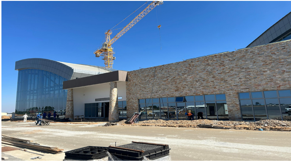
Robert Mugabe International Airport-New VVIP Pavilion
