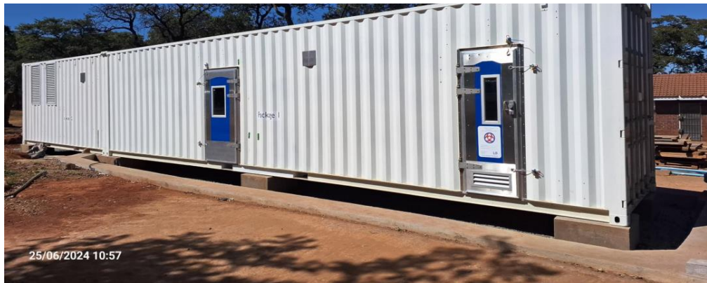
Sally Mugabe hospital containerised lab
