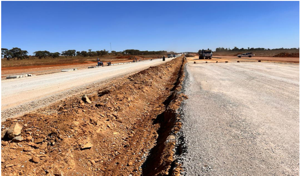
Bitumen World Road Construction Progress Base 1 level-Boulevard Road
