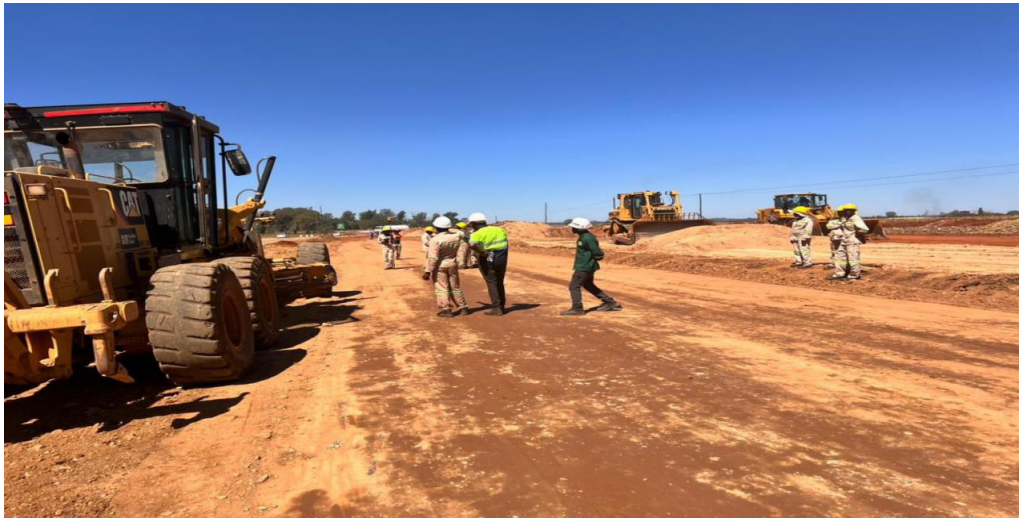
Exodus and Co, Harare-Mazowe Road earthworks construction
