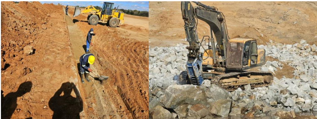
Construction of Kunzvi Dam in progress
