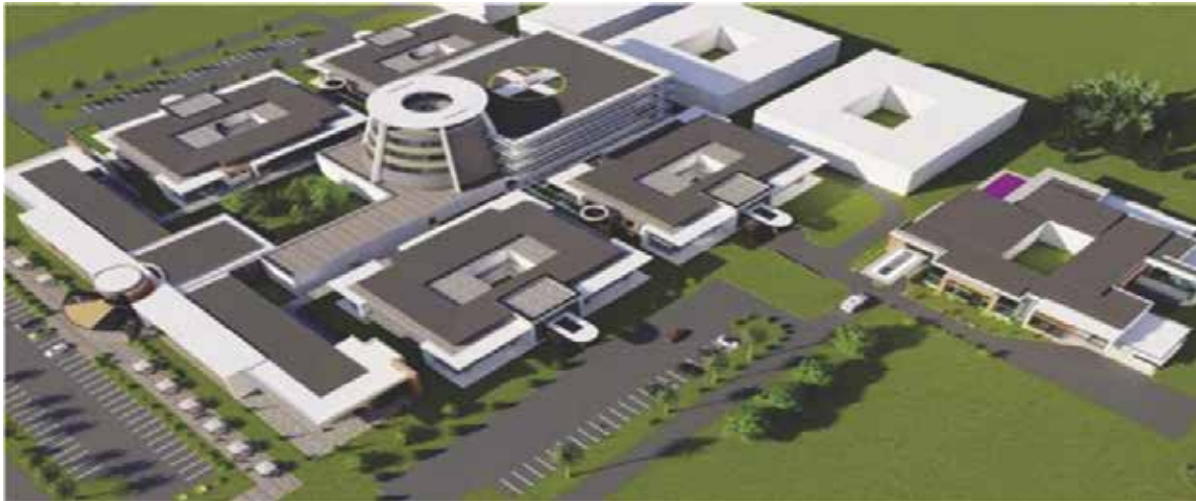
University of Zimbabwe Quinary Specialist Hospital Under Construction
