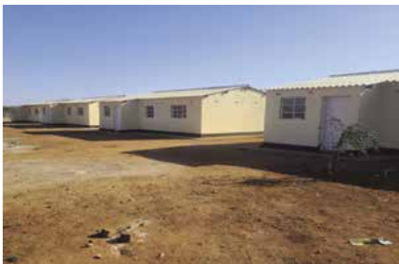
Mandihongola RHC Staff Houses, Gwanda RDC, Matabeleland South
