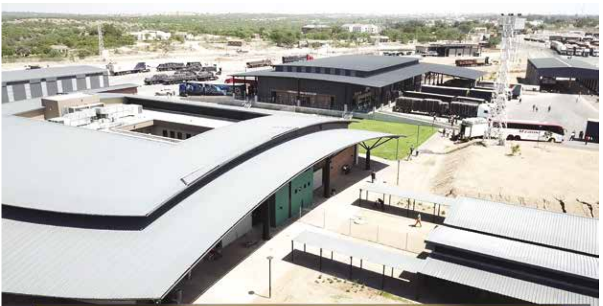
Upgrading of the Beitbridge Border Post enhances revenue collection and ease flow of people and traffic at the border
