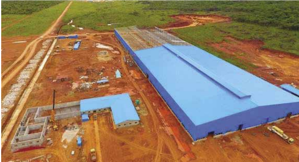
Construction of Manhize Iron & Steel Manufacturing Plant
