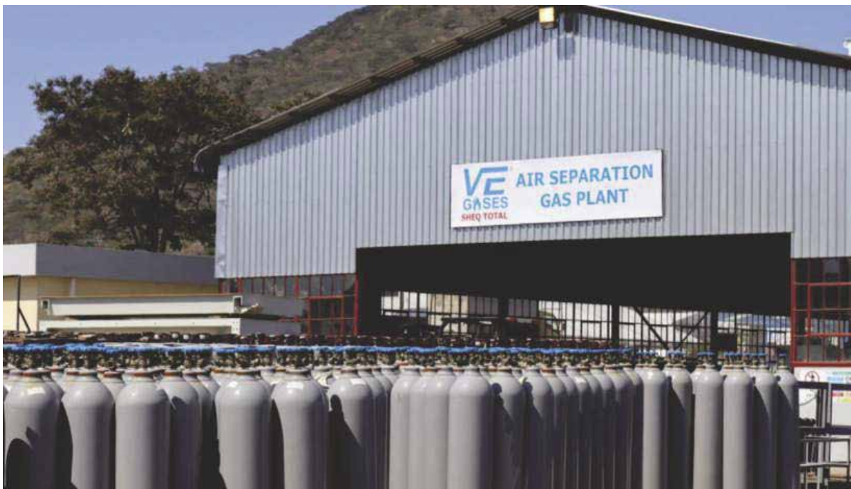
Constructed Medical Oxygen Production Plant
